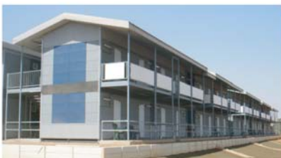
AUSTRALIA ; FMG PROJECT 720 MAN CAMP
